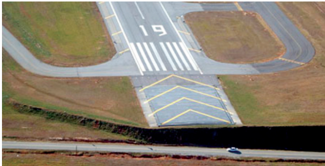
Figure 9.1—Photograph of an EMAS Installation
