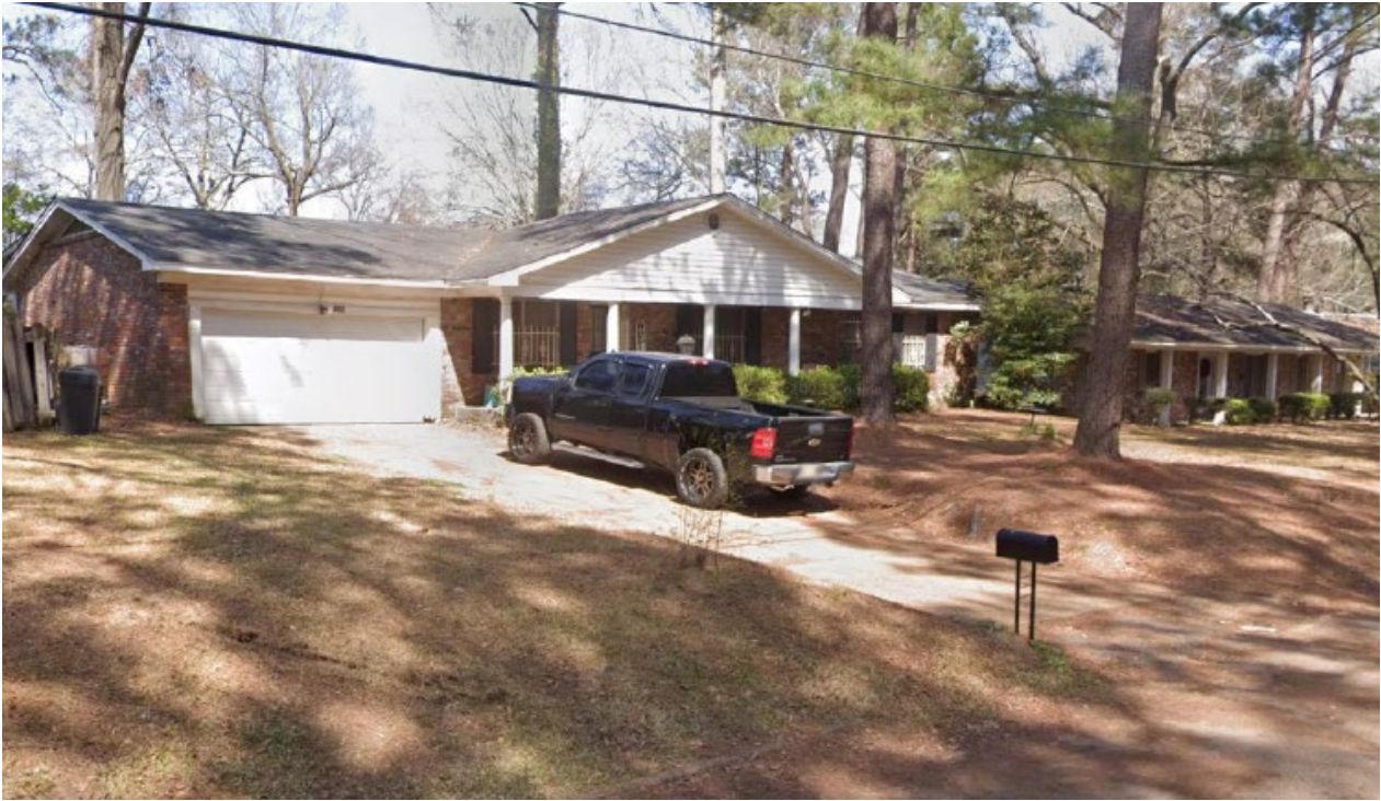
Figure 5. The Shalimar Drive accident home before the explosion. (Courtesy of Google Maps.)
