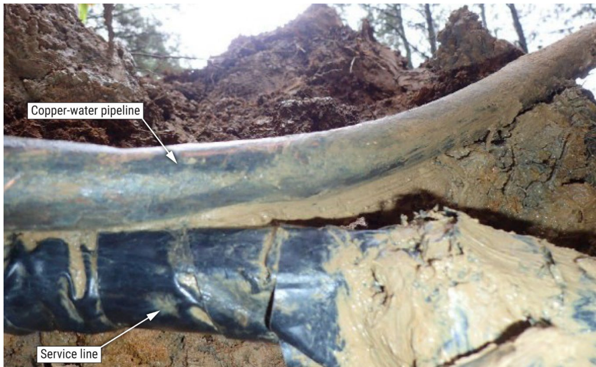
Figure 16. Excavation photograph of the copper-water pipeline and the service line near the Bristol Boulevard accident location. (Courtesy of Atmos.)
